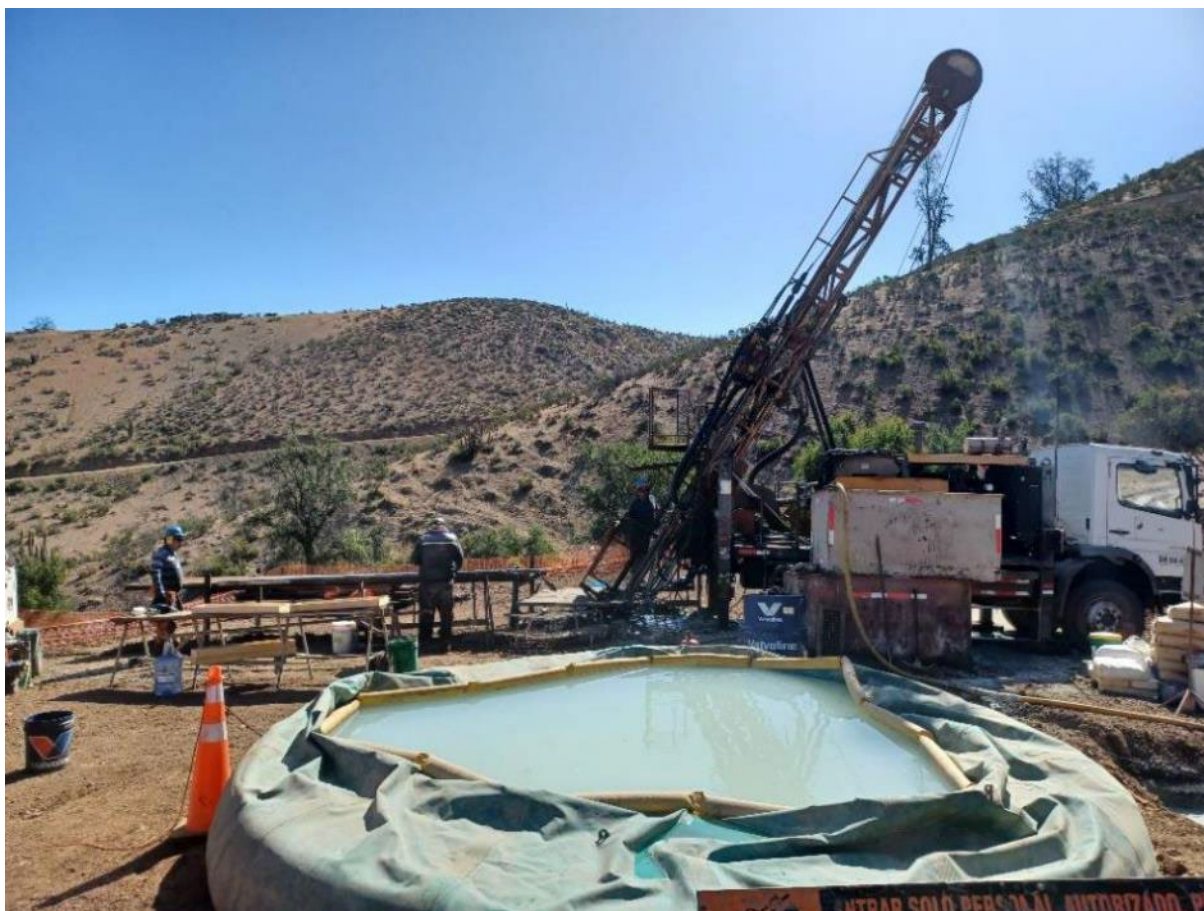
Figure 3: Drill rig positioned at drillhole collar CMQDD001 at the Anico prospect within the Quelon Project.
